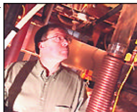
Mike Swinton demonstrates the Shower Heat Recovery System.
