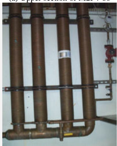
(c) GFX Model M2P4-60 Effectiveness: 72% (4.5 gpm balanced); 85% (4.5/6.5 gpm)
