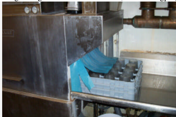
(d) Hobart dishwasher Models C-44A/C-44AW (Discharge: 5/2 gpm; capacity 203/126 racks/hr, respectively)
